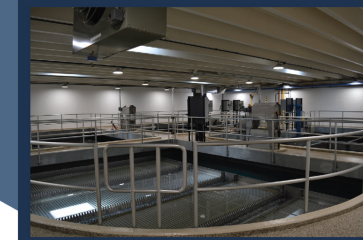
High-rate sedimentation system with inclined plate settlers
