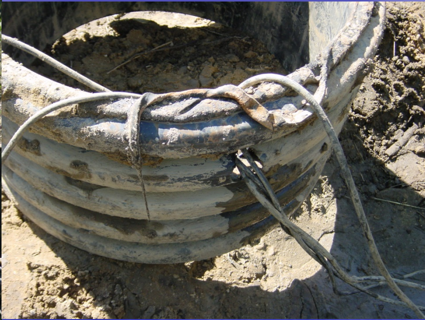
Pinched wires and sand intrusion.
