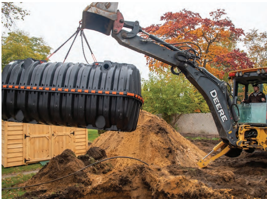
Travis Barrette operates a John Deere backhoe and lowers an IM Series tank from Infiltrator Water Technologies into the ground during a septic system installation.
